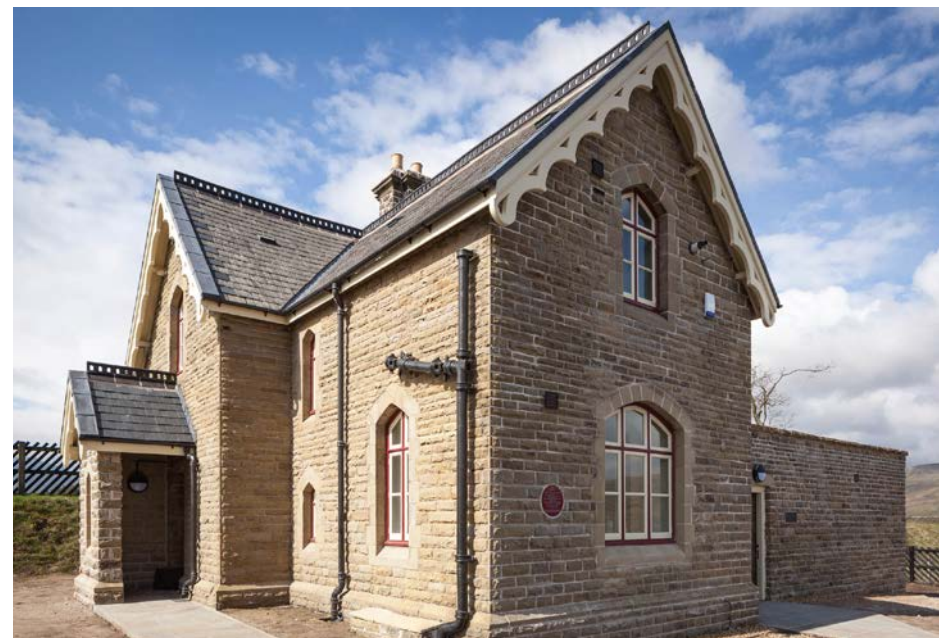
Ribbleshead Station Master's House. Photo courtesy of Railway Heritage Trust
